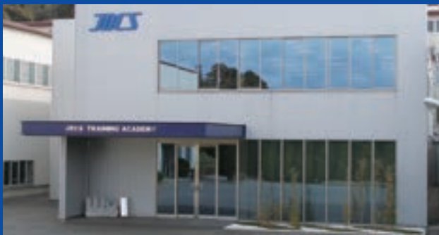
Training center adjacent to factory
