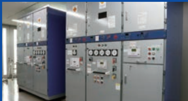
High-voltage switchboard simulator
