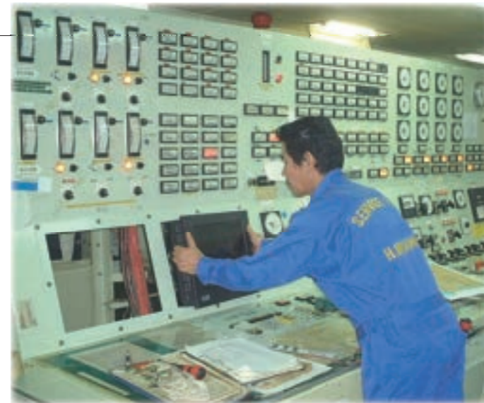
Alarm & Monitoring System Retrofitting Work (Engine Control Room)
