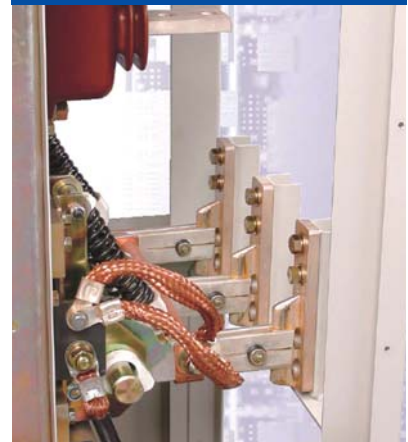
Closing Earthing Switch
