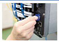
Control software updates and CSV data extraction (for viewing on PC) are easy thanks to built-in SD card support
